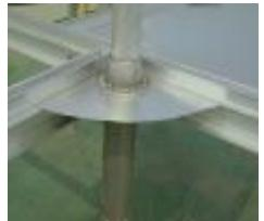
The Corner Connector (right) keys into the main I-Beam
