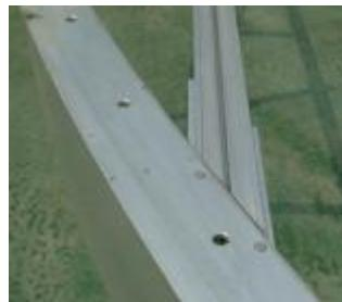
I-Beam to Rim bolted connection is strong and provides a clean surface for the sheeting and its clamping
